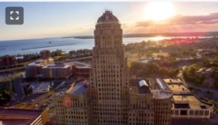
A view of downtown Buffalo, N.Y., and its art deco City Hall.
